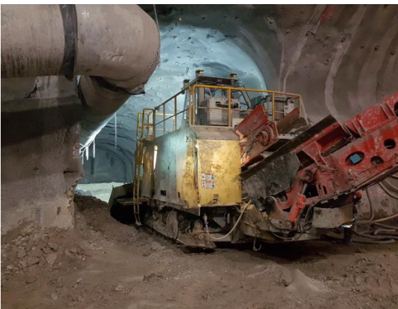
Benching - excavation of tunnel base
